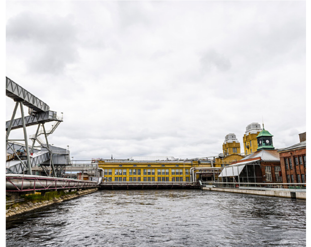
Water plays a central role in our production, heating, cooling, and cleaning processes.
